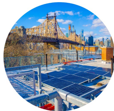
Solar roof installations at Queensbridge Houses
