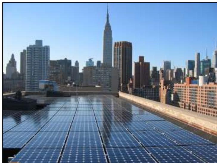
**Kips Bay Tower** in Manhattan: 20-story condominium building. 54.28 kilowatt solar system provides 57,000 kWh per year.
