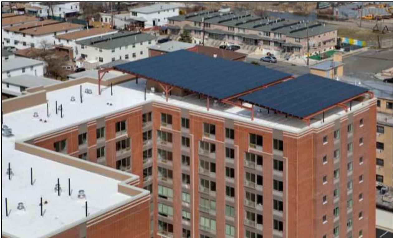
**Dumont Green** in East New York: 8-story, 176-unit, low-income rental building. 80.5 kilowatt solar system provides power to cover 80 percent of the laundry facilities, elevators, common areas, and security systems.
