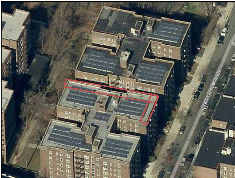
Example of required clear paths to comply with the NYC Fire Code. The red indicates clear paths on one section of the building but note that clear paths are required on each part of the “H”-shaped roof.
